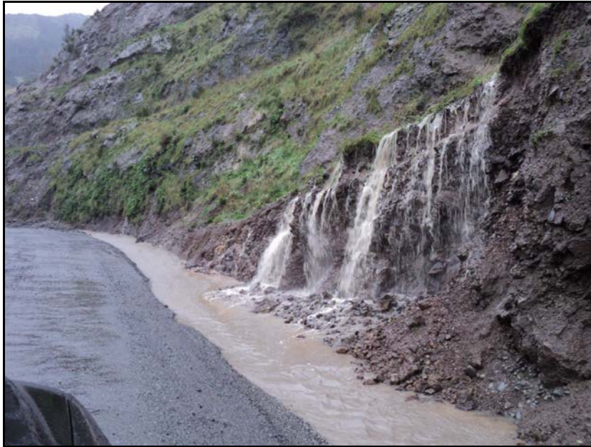
Photograph 1: Flooding adjacent to the existing haul road
