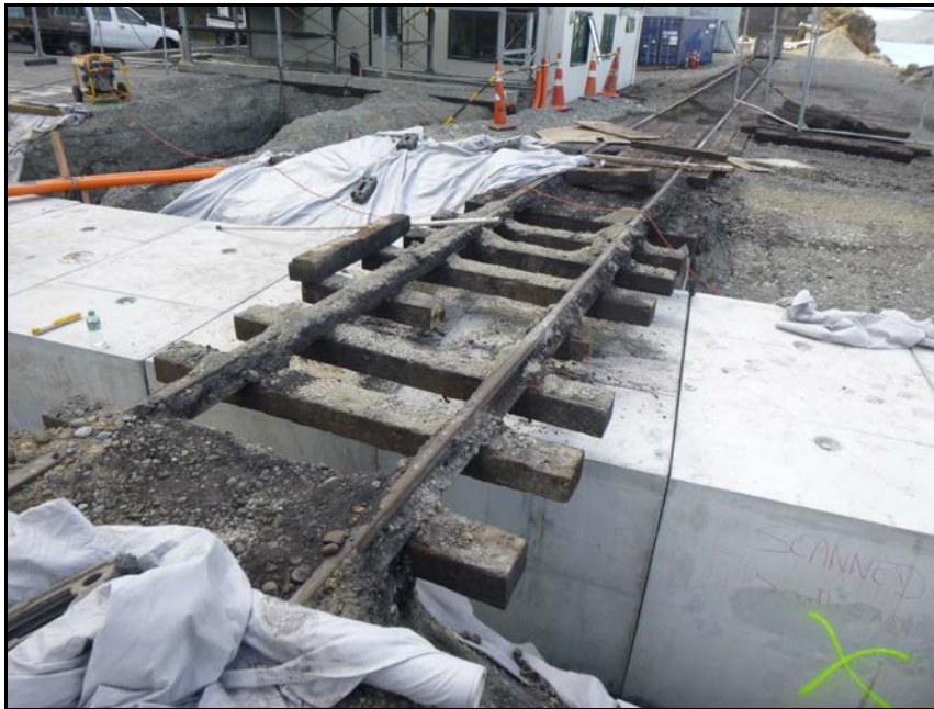
Photograph 3: Box culvert crossing under the existing railway
