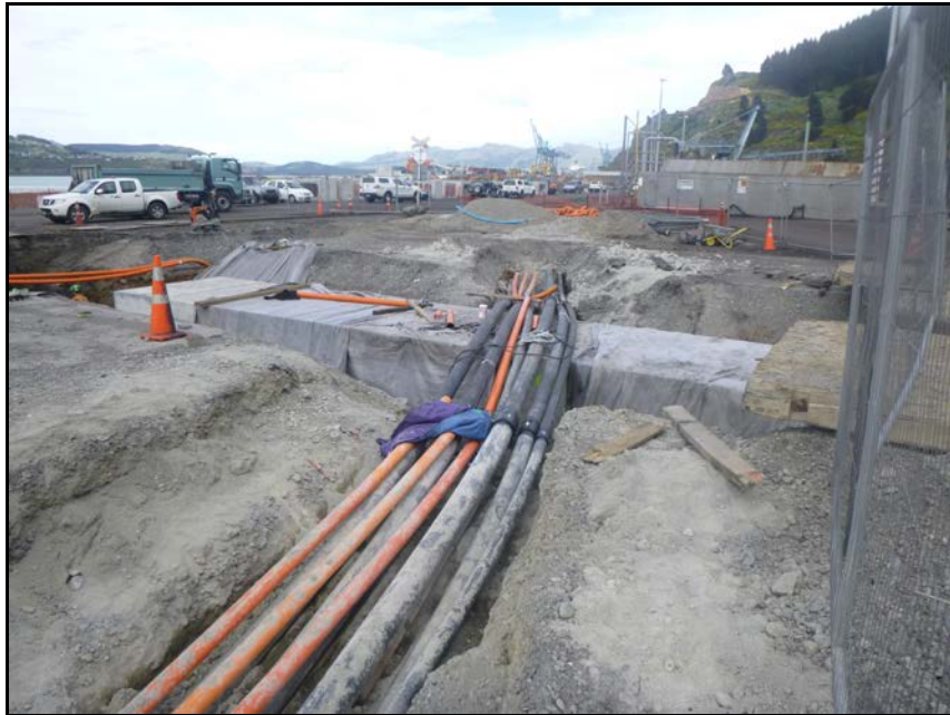
Photograph 4: Re-route of existing services over box culvert
