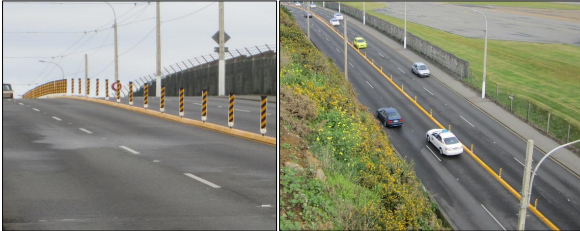
Photos 1 & 2: Separation kerb with flexible posts at completion
