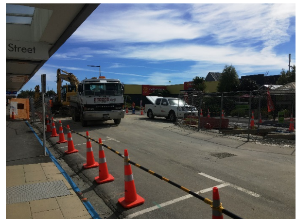
Figure 6: Construction Establishment in the ‘Blue’ Box
