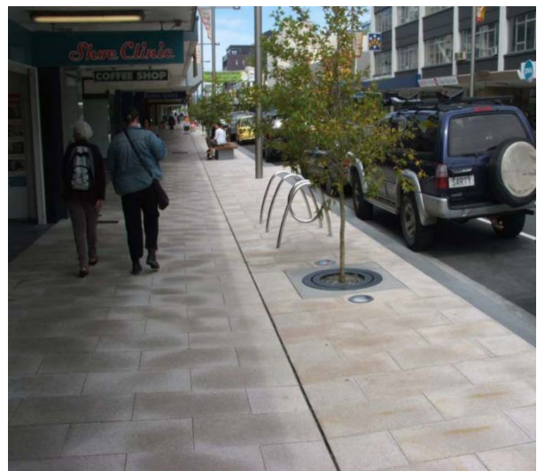
Figure 4: Inverted Crown in pavement (Another town)
